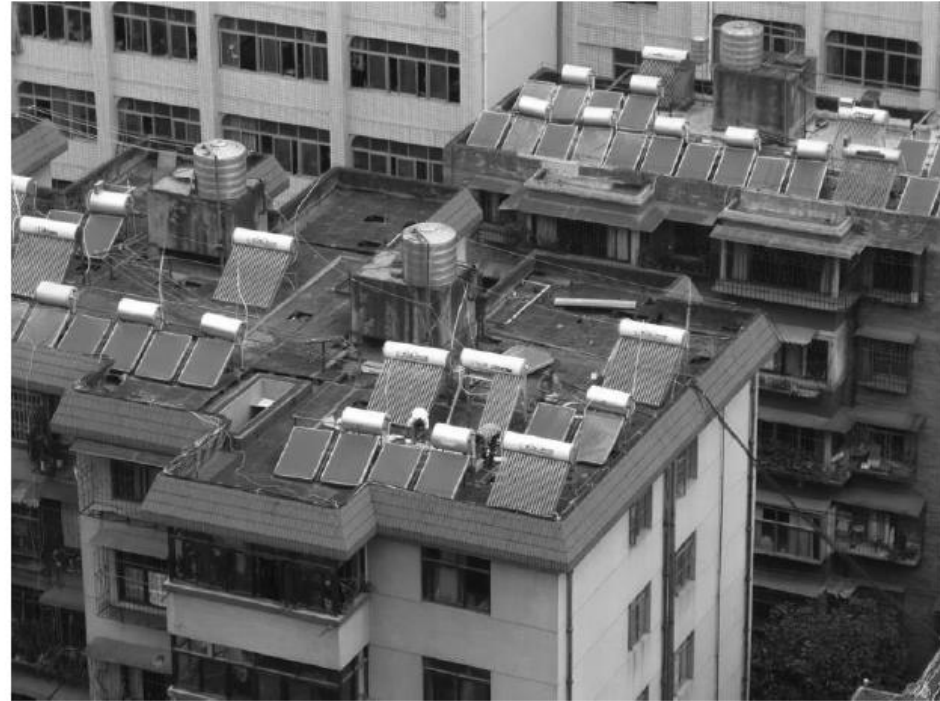
Fig. 5.3 Solar water heaters mounted on rooftops in China.
